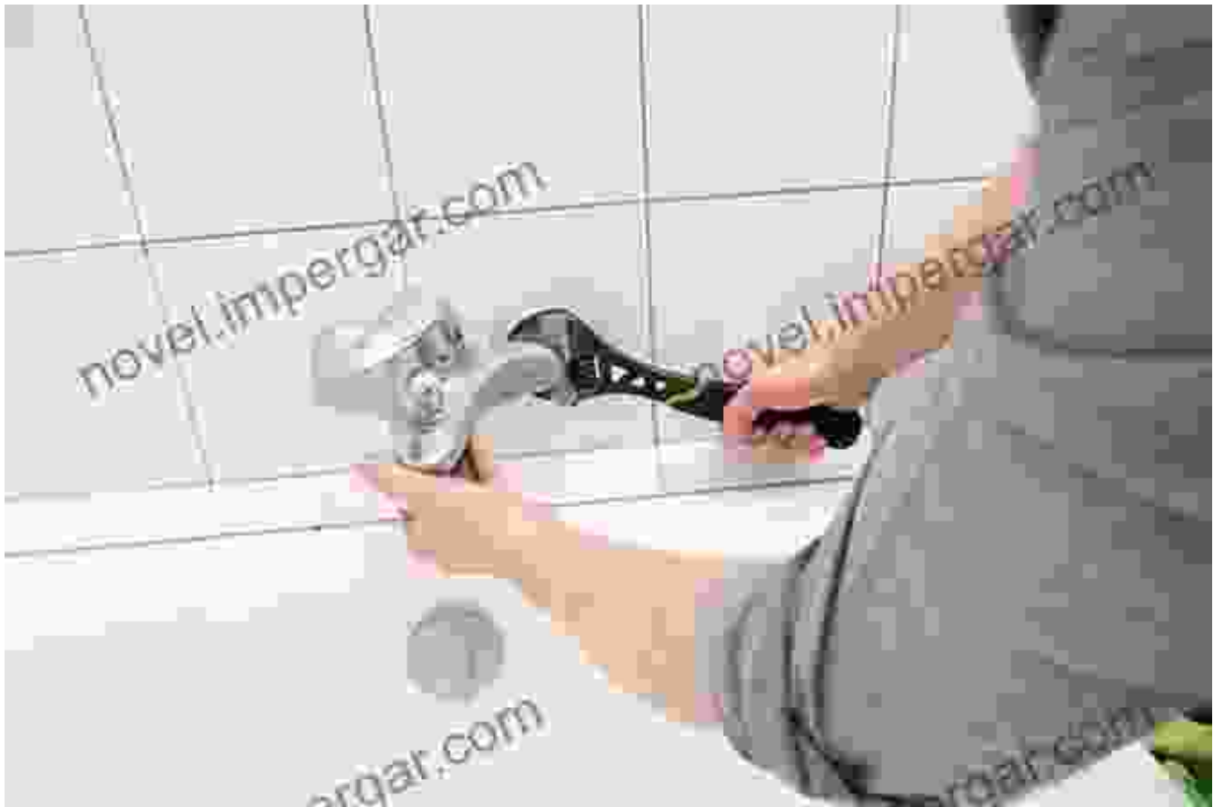
Figure 2: Repairing a Leaky Faucet
